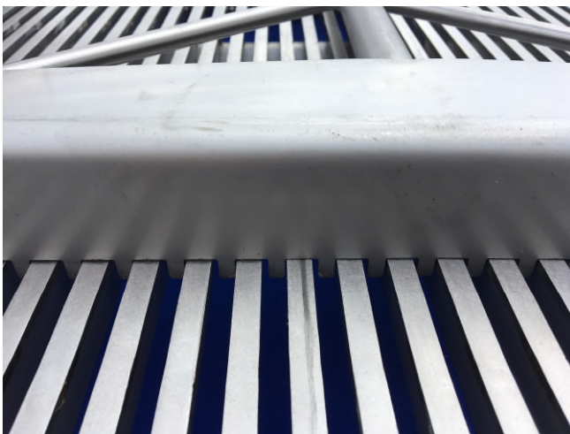
Manual Bar Screen in Tank
