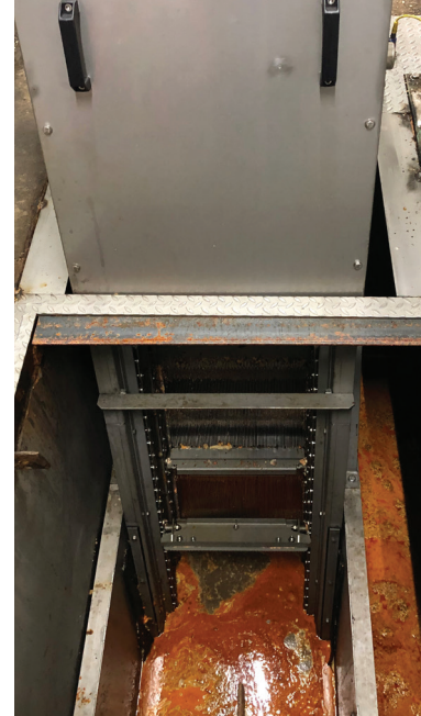
Blue Whale Micro Bar Screen with 2mm bar spacing in operation on high FOG food processing waste with TSS up to 10,000 mg/L
